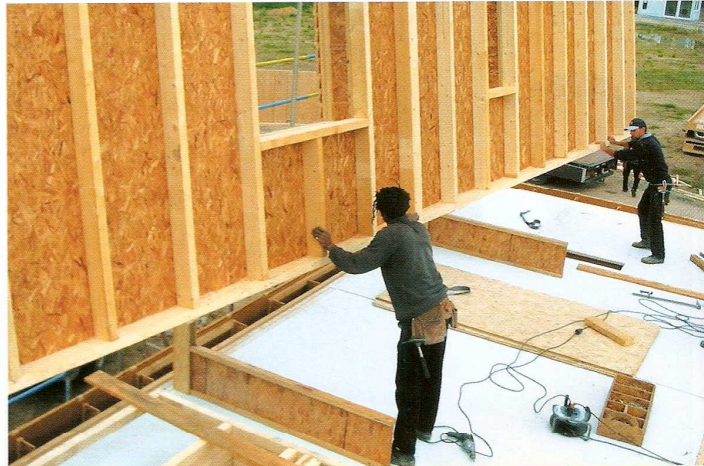
Prefabrication of wooden wall or roof elements under controlled condition can ensure a higher quality standard and a more rapid progress of work on the construction site: an economic advantage!
