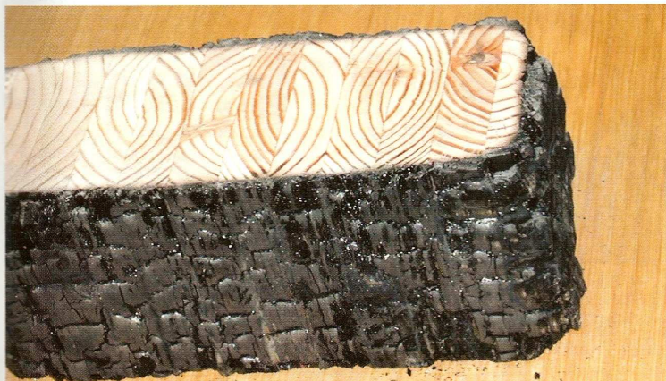
This cross-section of a gluelam beam is showing how the outer layer of charcoal prevents it from completely burning and collapsing. In addition you can nicely see how gluelam beam are made from several layers of quality boards.
