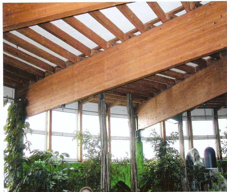
Glued laminated timber to support big roof constructions are being used more and more worldwide due to their economic, ecological and aesthetic advantages. Rising prices for steel and concrete are a good reason for Indian architects to think about this alternative as well.
